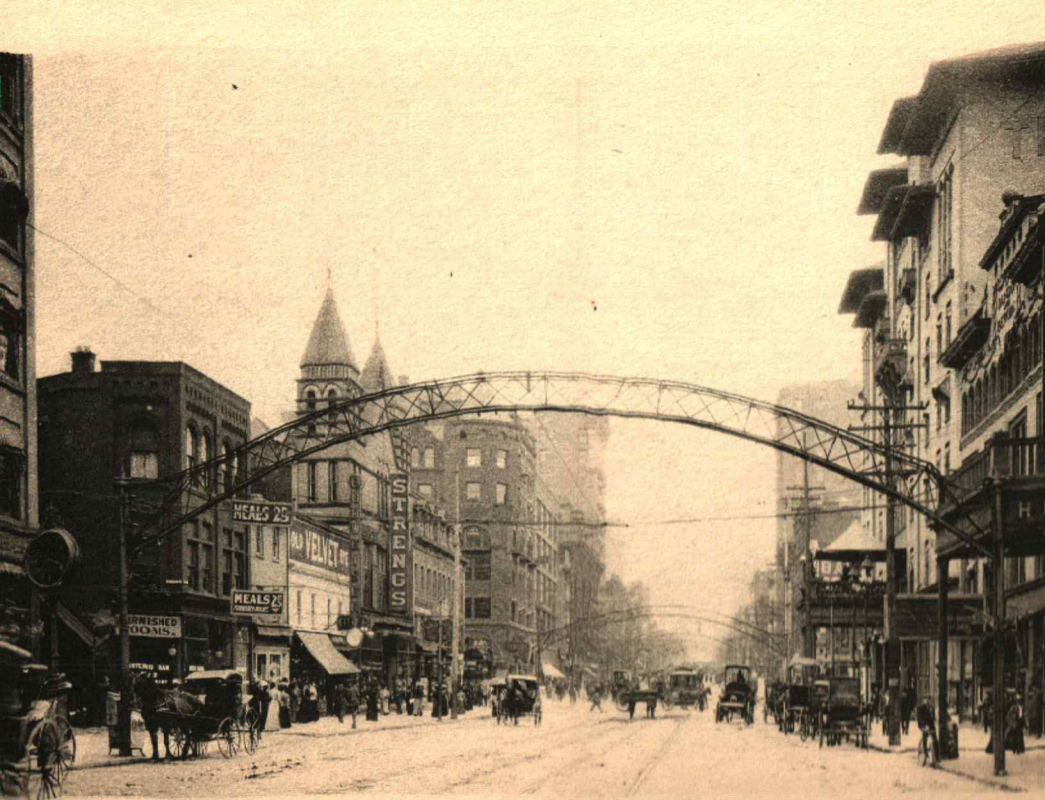
HIGH STREET, LOOKING SOUTH.
